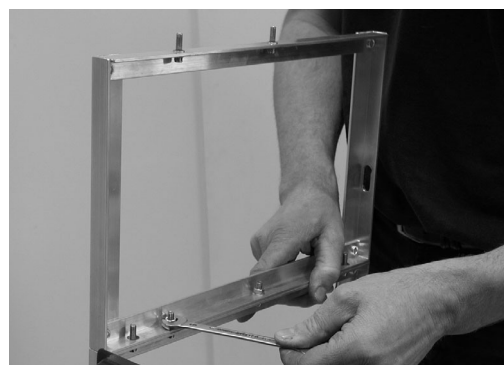
Montar as bases das consolas
